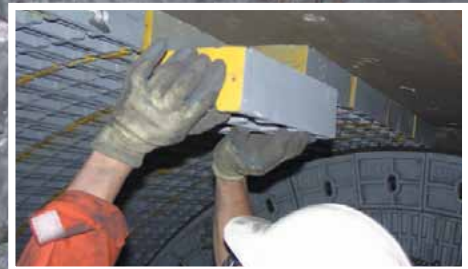
▲ A magnet holds the liner to the drum.
