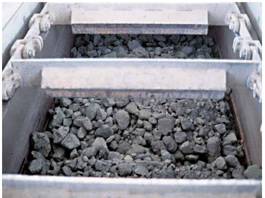
View into Chain Conveyor – Limestone feeding
