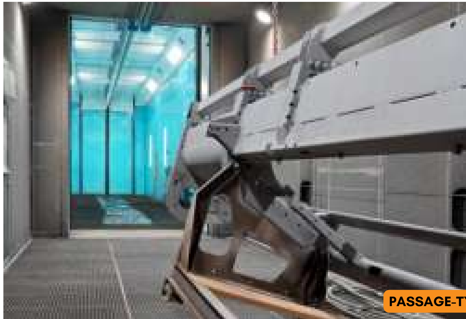
Travel from the blast room into the paint spraying booth
