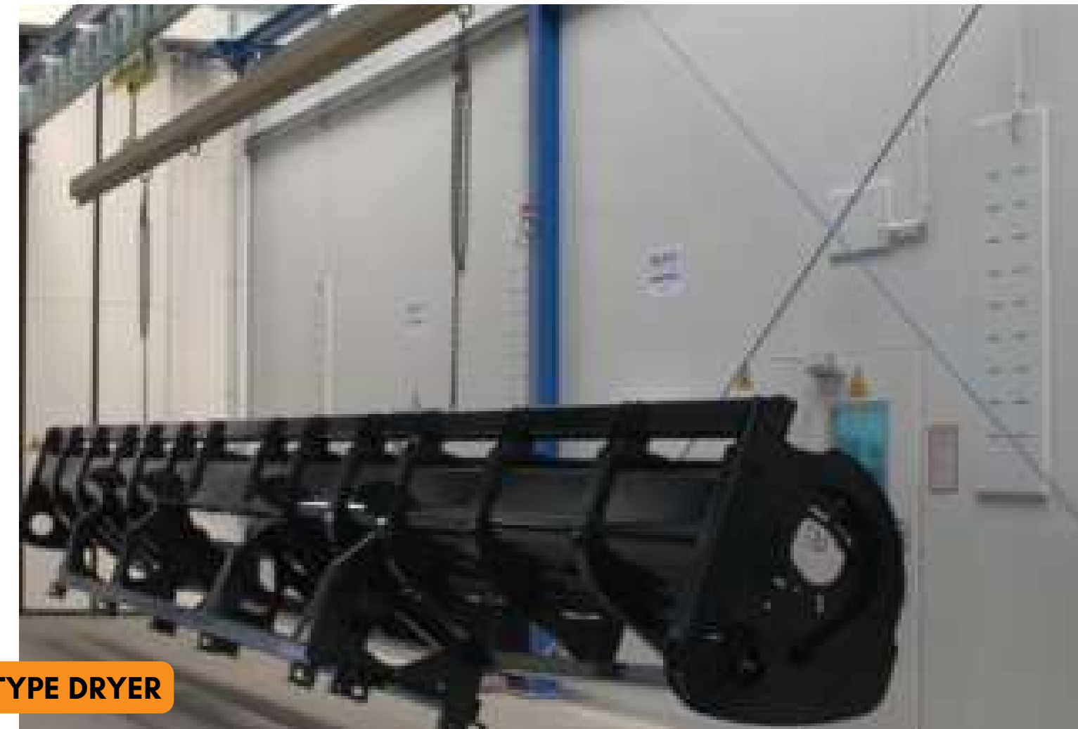
Cooling zone behind the passage-type dryer
