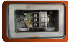
Terminal in separate compartment for safety
