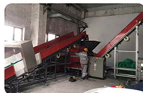
Material: Plastic Waste Solutions: Shredder+Washing Area: DUBAI
