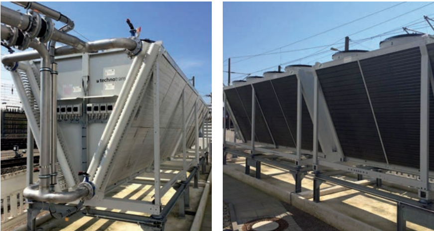
➤ technotrans recooling system: installation of several recooling systems for a large-scale railway project
