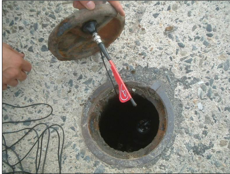
Fig. 55 Extension Antenna fitted to chamber lid
