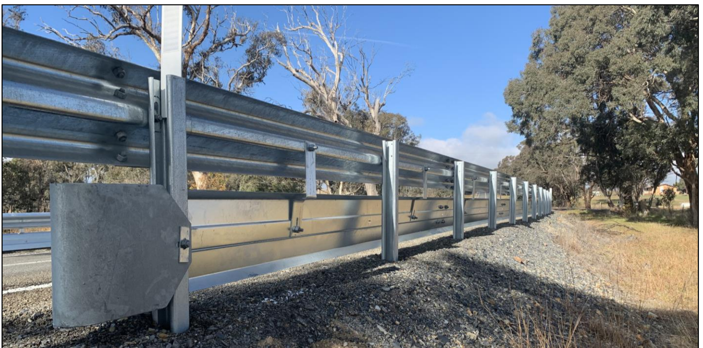
Figure 5: Attachment of Bullnose (rear views)
