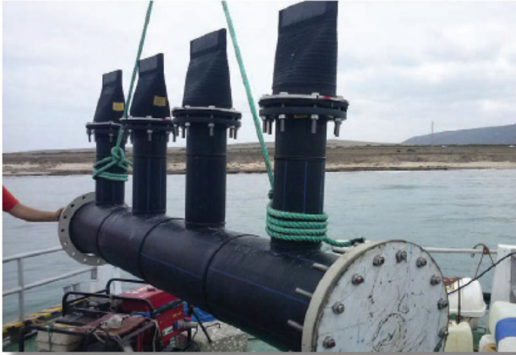
Detail of the ProFlex™ Flanged Rubber Check Valve; Style 710
