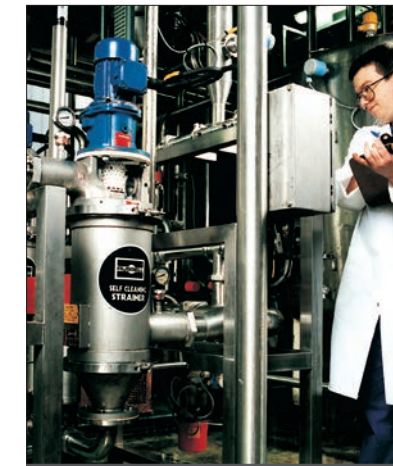
Self-Cleaning Russell Eco Filters® provide pre-filtration at a factory of H.P. Bulmer - Cider manufacturers
