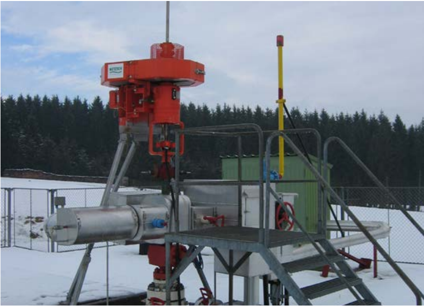
Pump in a methane application with optional remote well monitoring and control
