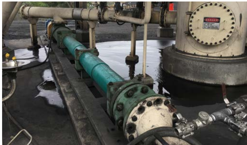
Excellent solids handling and pressure capabilities enable the handling of demanding slurries with NEMO® progressing cavity pumps.
