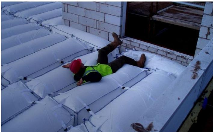
Falling from even a small height can cause serious injury, that's why having the right fall arrest systems in place is so important. Inflatable airbags from AirDeck provide an easily transportable fall arrest solution.
