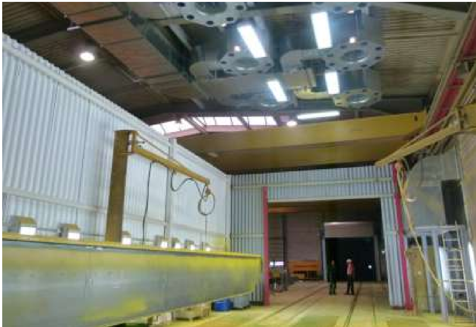
Reconstruction of the existing supply air system of the paint spraying system to long-range nozzle technique
