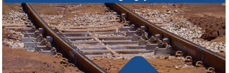
Installation of INFINITY 'LS' weighing system in curved track
