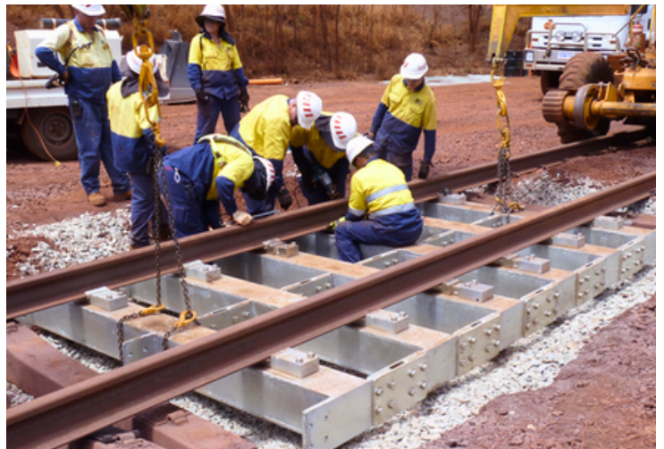
Installation of INFINITY 'LS' weighing system in curved track
