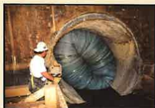
Inserted liner for repair
