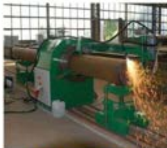
PIPE ROTATORS AND PIPE WELDING
