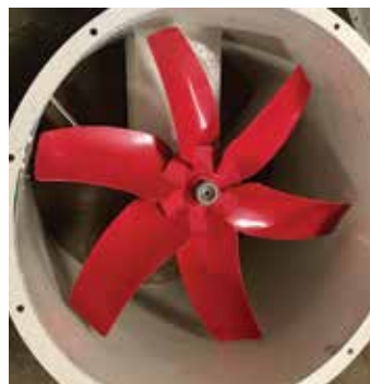
EXE Axial Flow Fan used on a spray booth project
