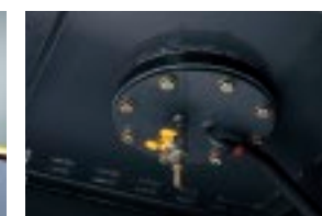
Maintenance hole for cleaning
