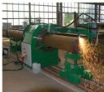
PIPE ROTATORS AND PIPE WELDING
