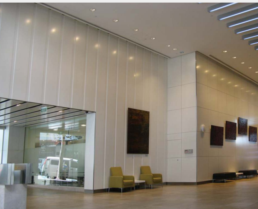
▼ SUPA COLOUR panels form a durable and attractive entry to a city building with extra wide joints and matching backing strips.
