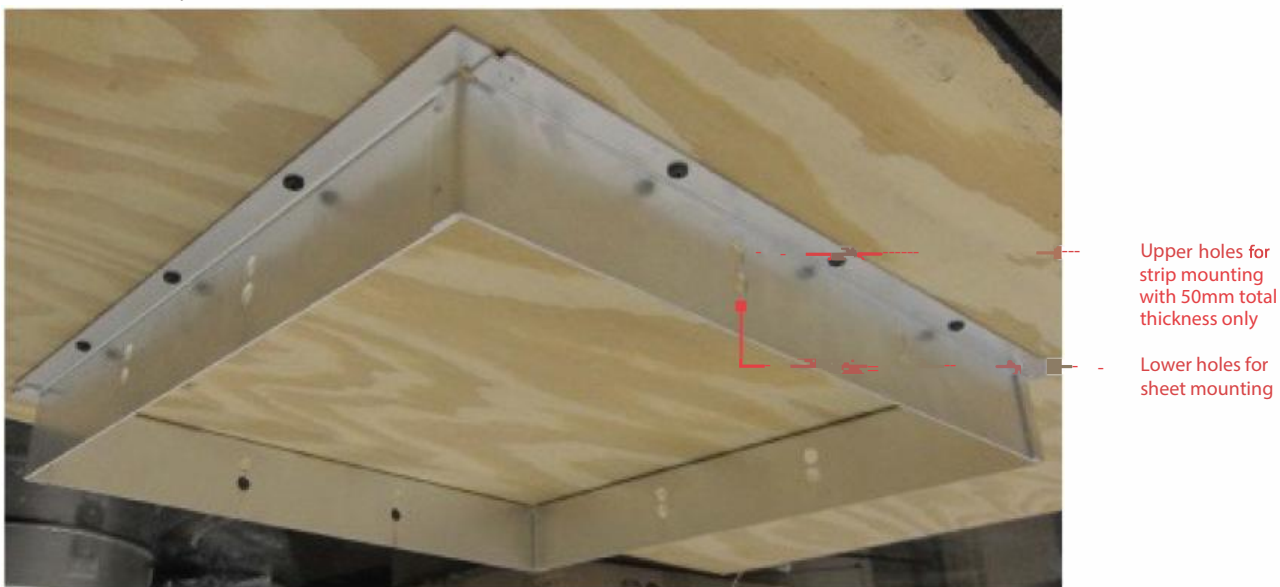
Figure 5: Incogneeto Frame Mounted Onto Plywood Sheet
