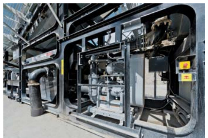
Centrifugal Pumps, Roll out for Service Access
