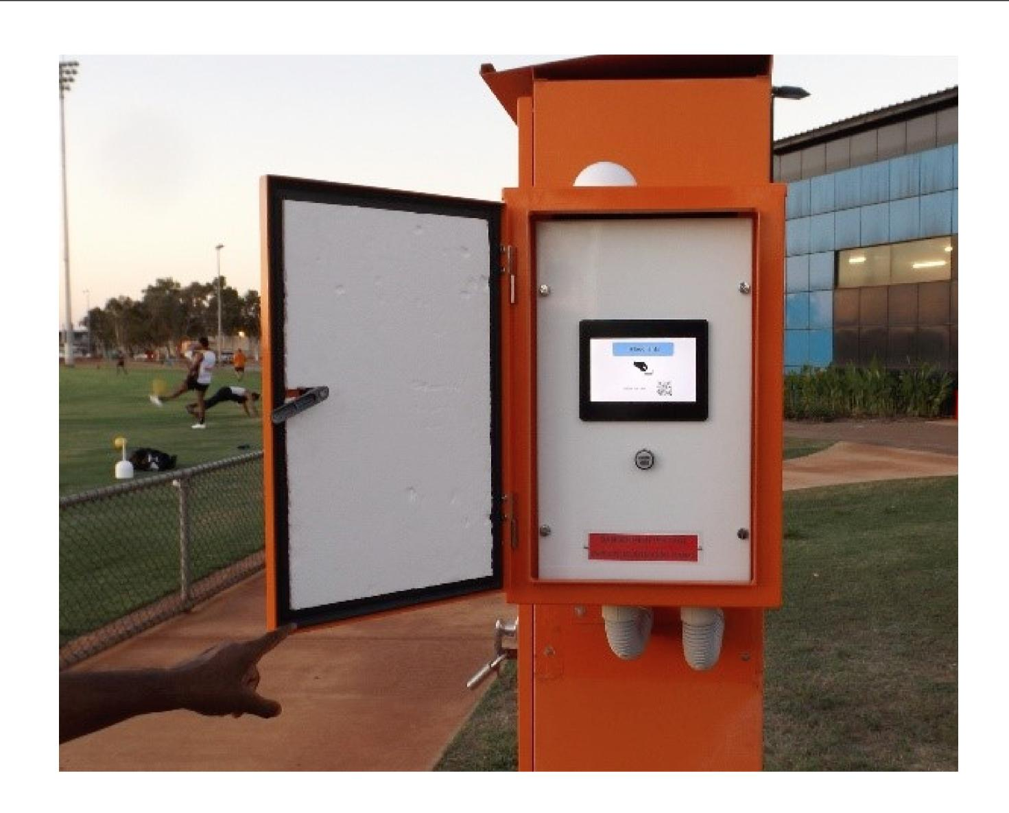
Floodlights use a lot of energy and for most installations there is no incentive to be more prudent in using the lights. The Smarter Floodlight Control System provides swipe card and mobile device access for individual control of poles and lamps.
