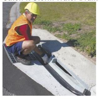
The Catch-it is a robust stormwater drain pollution protection system. Made from solid durable recycled plastic and rubber components, it can be moved from site to site. It is designed for road-side or side entry drains and reduces the amount of sediment or solid pollution entering the drain from the side.
