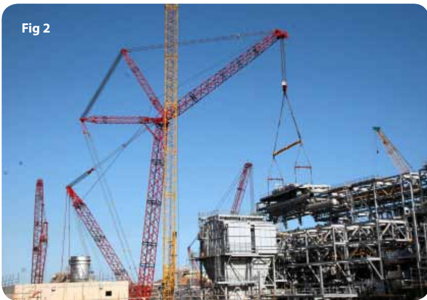
Fig 2: '1 over 2' rig formation used in Oil Refinery building project
