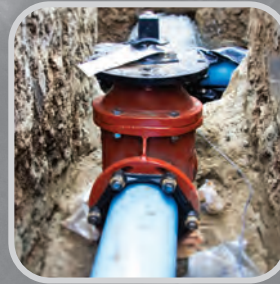
Water and Sewer Lines
