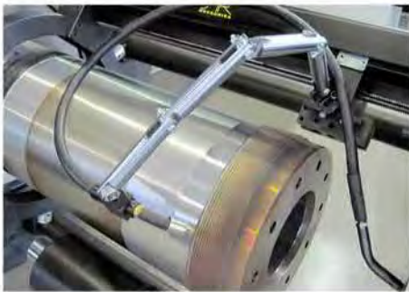
External Overlay welding
