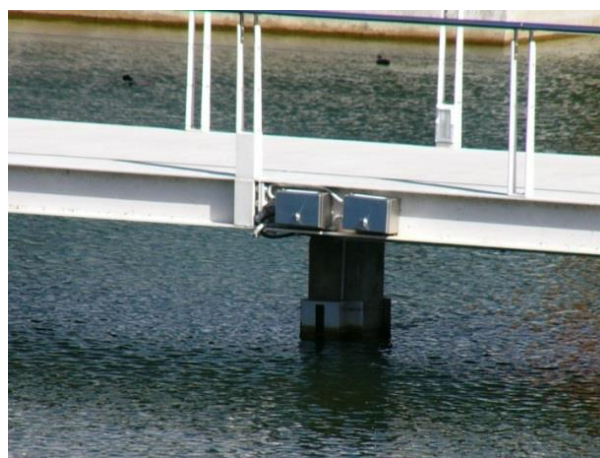
Algae controllers unobtrusively installed below the foot bridge
