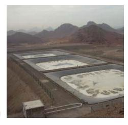
accordingly. The pipe work should be in metal, if plastic pipe is used, then the first 6 meters of pipe work should be metal in order to bring the air temperature down to at least 90 °C in the plastic pipe. In lakes and lagoons, make an air ring main and come off the ring main with ½" flexible hose, fit a diffuser on the end of the hose, and then simply drop the diffuser into the tank. Installation is therefore simple and very quick.
