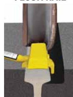
encased in pavement with only a flangeway on inside of rail
