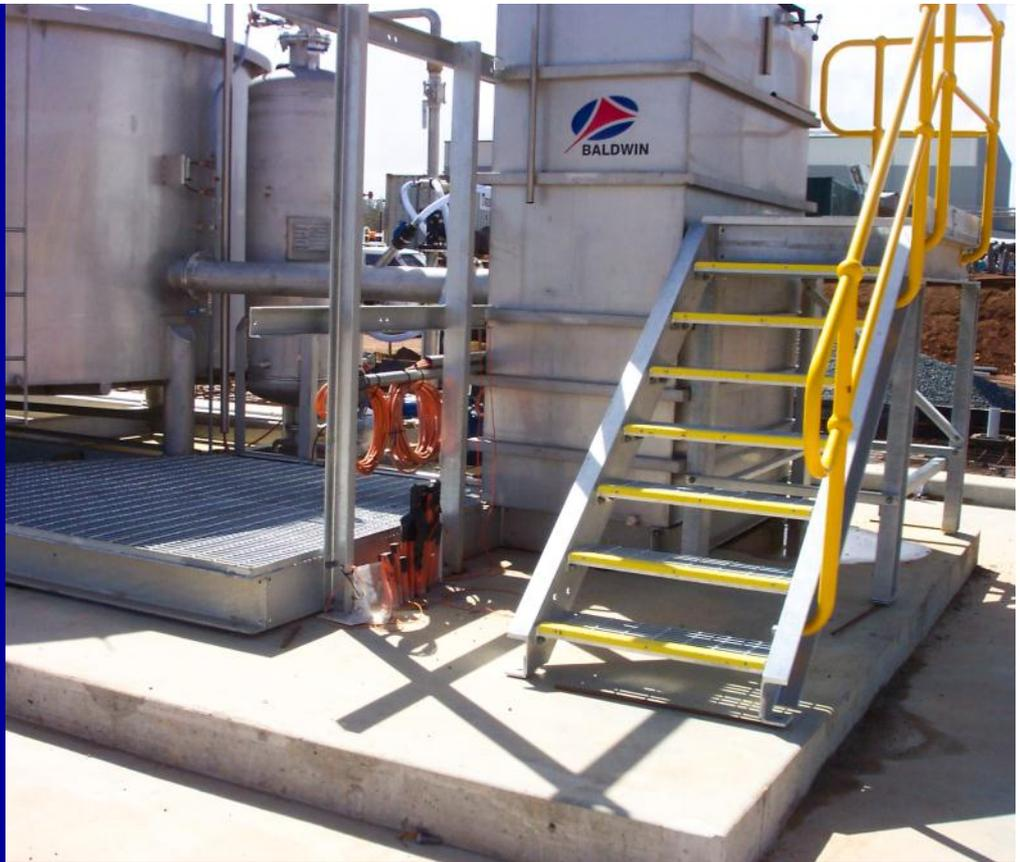
40,000L/Hr PLC Controlled Mine Site DAF
