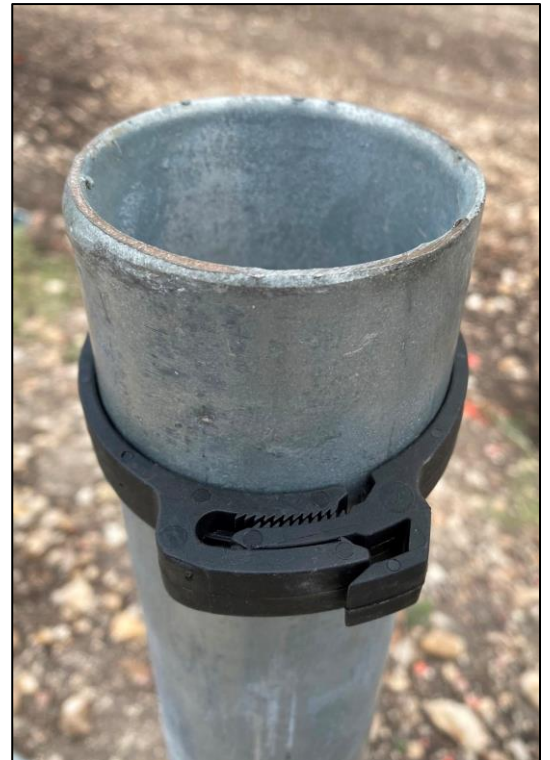
Figure 9: Securing of Retainer Clip
