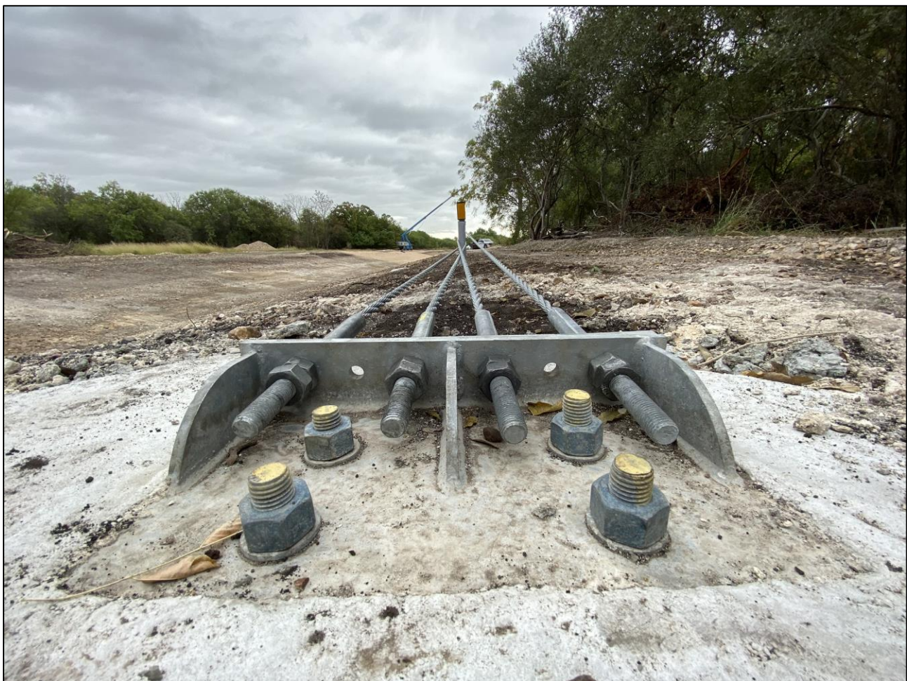
Figure 12: Anchor Bracket Assembly
