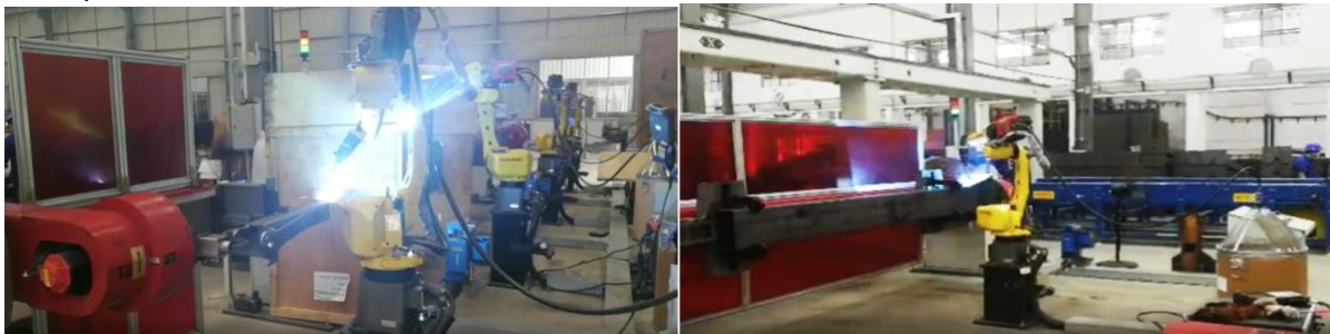
Figure: Arm and column welding of HAPP products.
